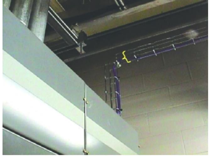
7. Due digital. A recent study concluded that outfitting a new power plant with all-digital controls would reduce instrumentation and control construction costs, by slashing outlays for installation labor and materials. Included in the study was a comparison of a typical cable and tray installation (left) with a digital network cable installation (right). Courtesy: Emerson Process Solutions
