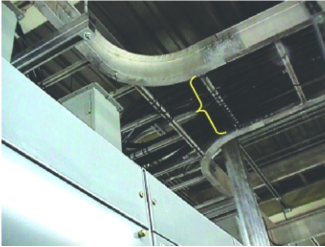
7. Due digital. A recent study concluded that outfitting a new power plant with all-digital controls would reduce instrumentation and control construction costs, by slashing outlays for installation labor and materials. Included in the study was a comparison of a typical cable and tray installation (left) with a digital network cable installation (right). Courtesy: Emerson Process Solutions
