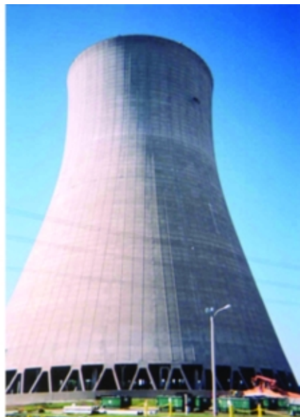
1. Elegant but exposed. The concrete and steel in counterflow (left) and crossflow (right) natural-draft hyperbolic cooling towers are vulnerable to corrosion-induced deterioration. Source: Structural Preservation Systems Inc.
