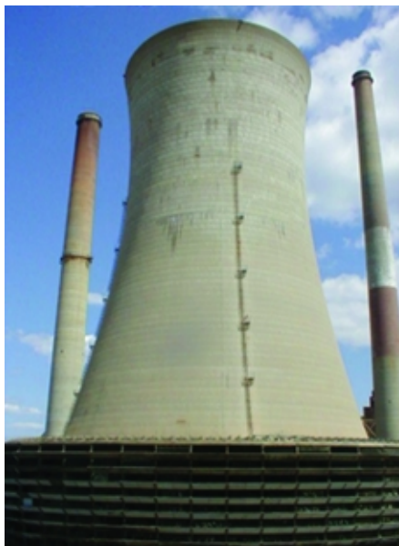
1. Elegant but exposed. The concrete and steel in counterflow (left) and crossflow (right) natural-draft hyperbolic cooling towers are vulnerable to corrosion-induced deterioration. Source: Structural Preservation Systems Inc.
